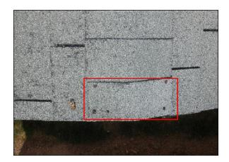
1.1 The metal flashing is mastic covered, monitor this area periodically for possible leaks at most vent type flashings rear side of home.
